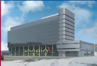
05/2008 Start of construction for the angelo in Ekaterinburg
